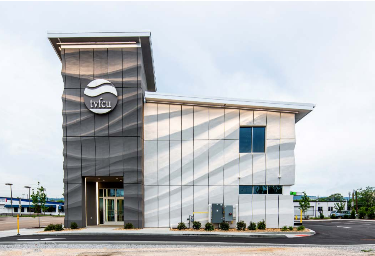
Branch's 3D print process enables it to create visually interesting building parts, such as the façade of this bank in Chattanooga, Tennessee. Credit: Branch Technology Inc.
