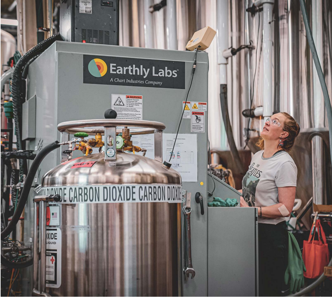
A brewer makes adjustments to the Earthly Labs carbon-capture unit, which purifies carbon dioxide from the beer brewing process for use in carbonation. Credit: Chart Industries Inc.
