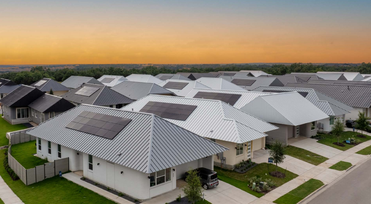
ICON built Wolf Ranch, the world's largest neighborhood of 3D printed houses, in Georgetown, Texas. The company worked in collaboration with homebuilder Lennar, which handled the roofing and finishings. Credit: ICON Technology Inc.
